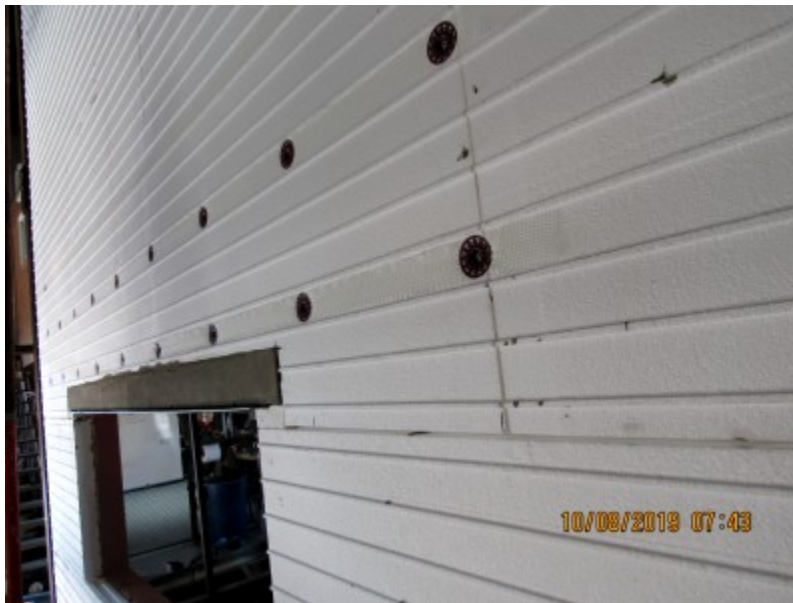
Photo No. 8 Fastener Installation Through Panels
