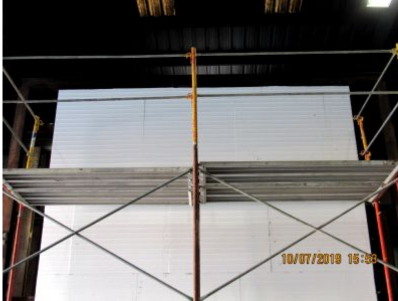
Photo No. 7 EPS Installed Over Wall
