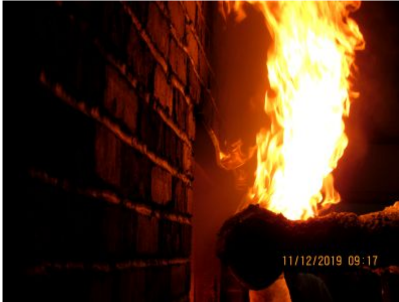
Photo No. 19 Window Header Flaming
