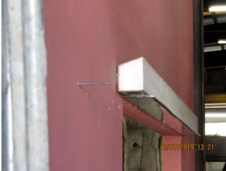
Photo No. 5 Window Detail With EPS
