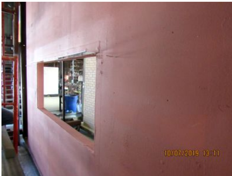
Photo No. 2 Base Wall with WRB and Window Header
