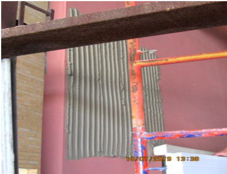
Photo No. 6 Stucco for EPS Installation
