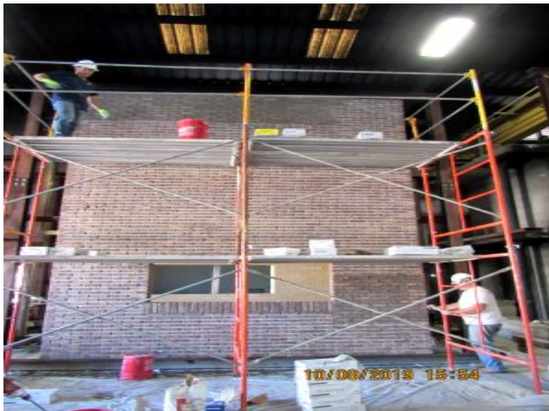
Photo No. 12 Brick Veneer Installed
