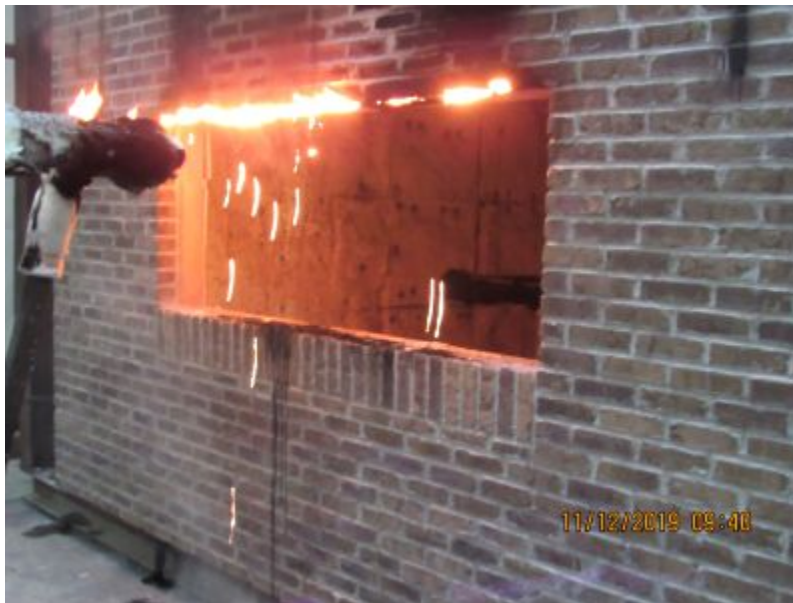
Photo No. 24 Post-Test
