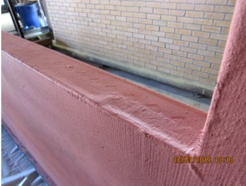
Photo No. 3 WRB Around Window
