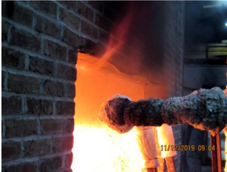
Photo No. 15 Window Header Sagging
