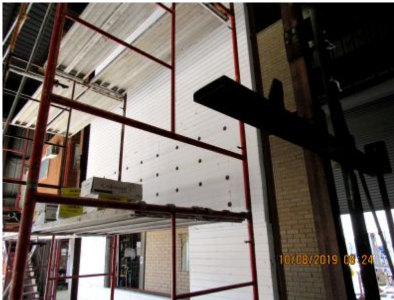
Photo No. 10 Fastener Installation
