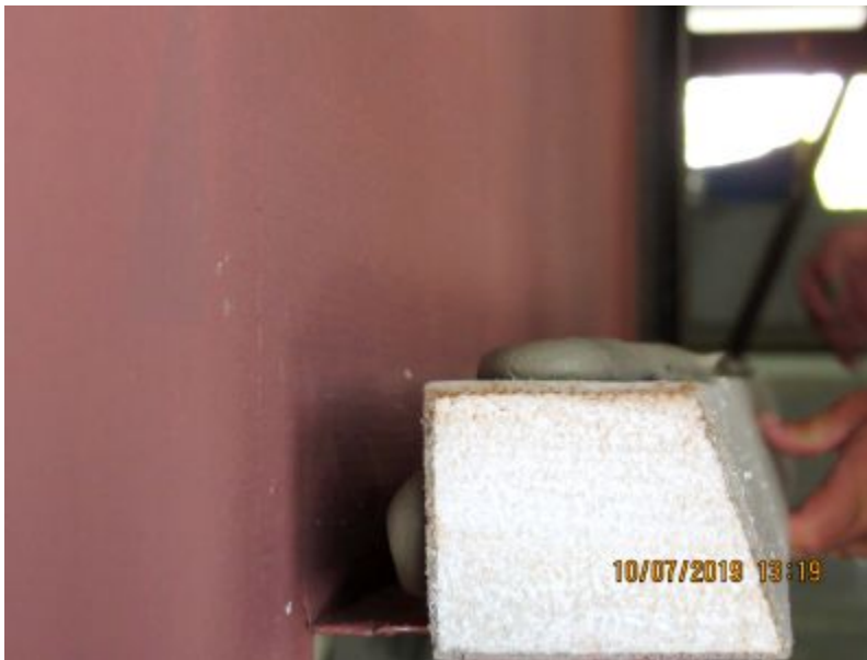
Photo No. 4 EPS Application
