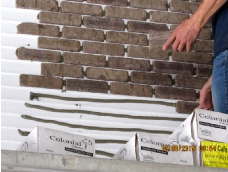
Photo No. 11 Brick Veneer Installation
