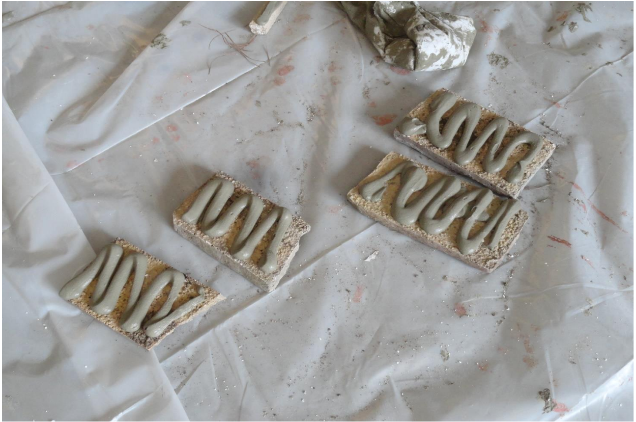
STONE VENEER WITH OLD MILL BRICK & PANEL ADHESIVE ON BACK SIDE
