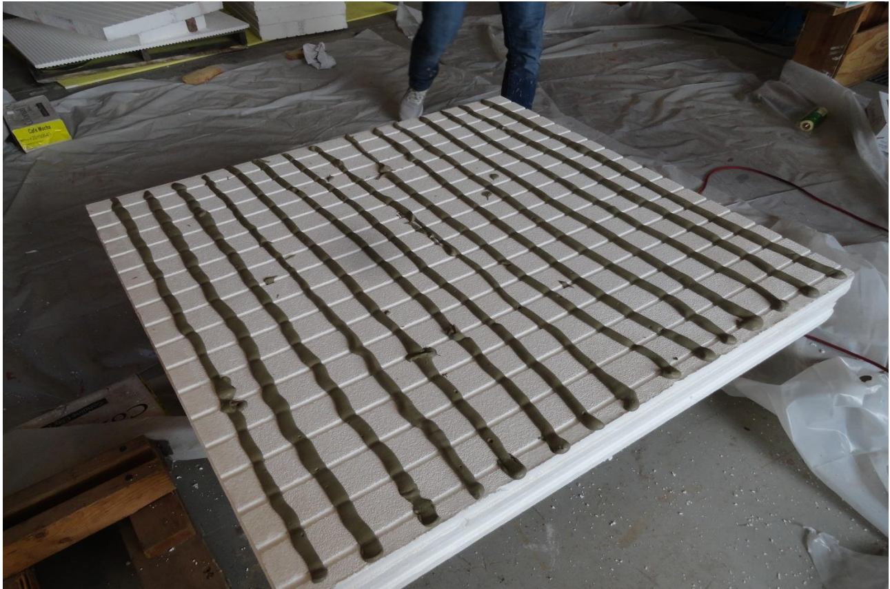
2"-3" O.C. ROWS OF ¾" BEAD OLD MILL BRICK & PANEL ADHESIVE ON BACK SIDE OF 3" THICK OLD MILL PANEL+ EPS FOAM
