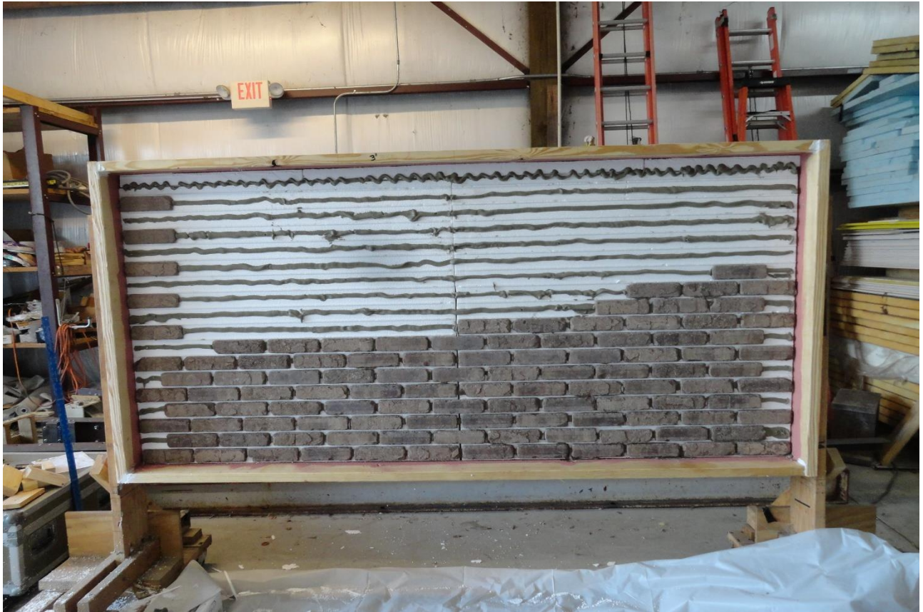
THIN BRICK INSTALLED INTO HORIZONTAL \frac{3}{4} " BEAD OF OLD MILL BRICK & PANEL ADHESIVE
