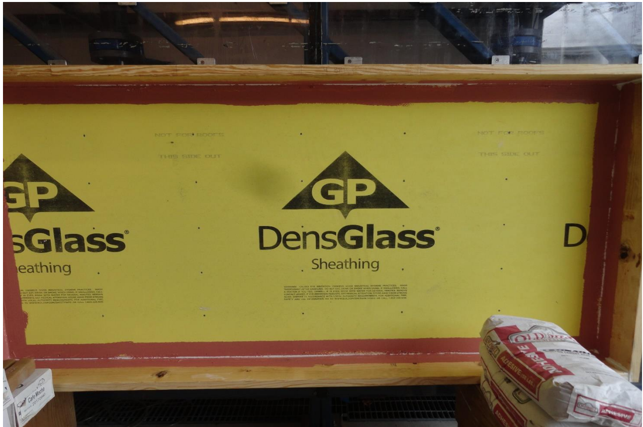
½" DENSGLOSS SHEATHING FASTENED TO STEEL FRAMING
